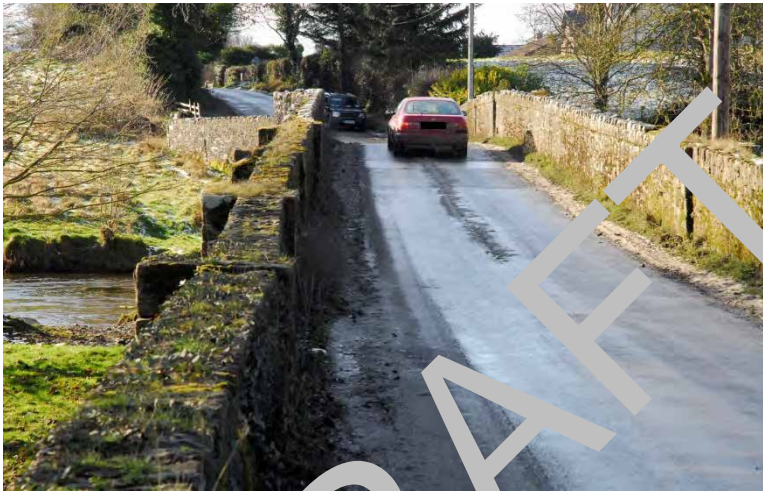
Plate 7. View of car crossing Donaghpatrick Bridge
